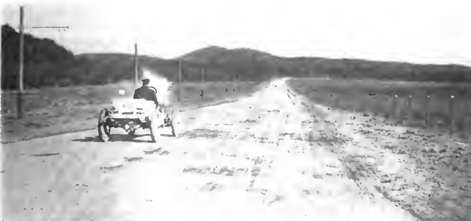
Sloat Boulevard, Recently Completed, Without a Bump in It
